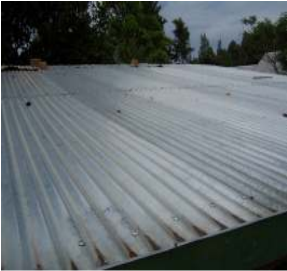
Figure 5 Roof of the underground tank
