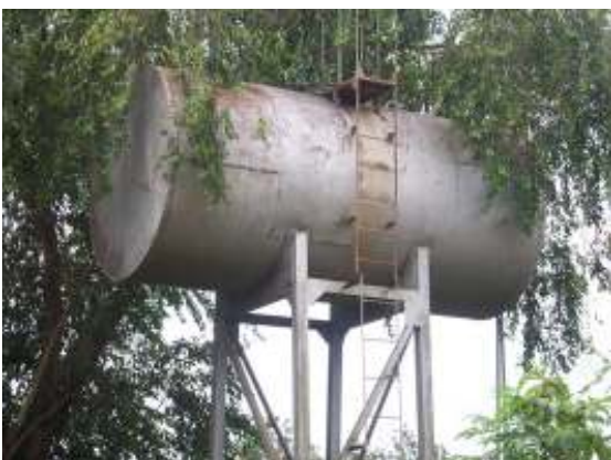
Figure 7: Tank used for irrigation
