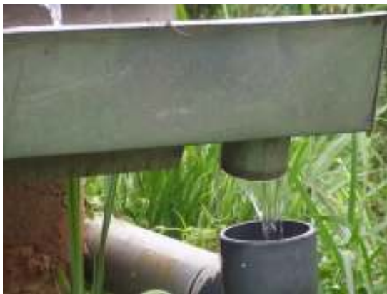
Figure 6: Water flowing from the tank
