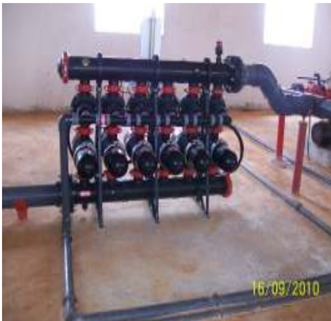
Figure 2: Filter machine for drip irrigation
